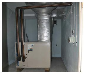
Figure 1: Evaporative component of the air handling unit, commonly referred to as the 'air handler'. This is usually located within an air-handling room.
