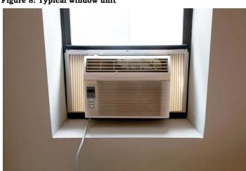
Window units have all of the components housed in one box. Window units tend to be noisy because the compressor *(which is a part of the condenser)* is noisy.
