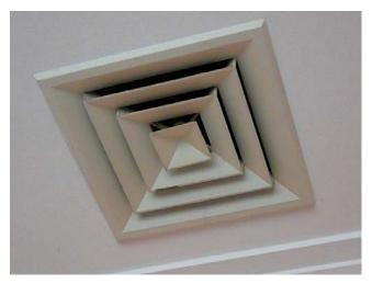
Figure 4: Typical diffuser vent
